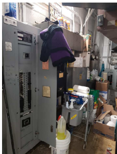
Open panel and housekeeping hazards
